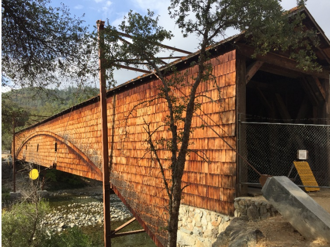
Figure 3: Bridgeport Bridge with Temporary Stabilization Frame
